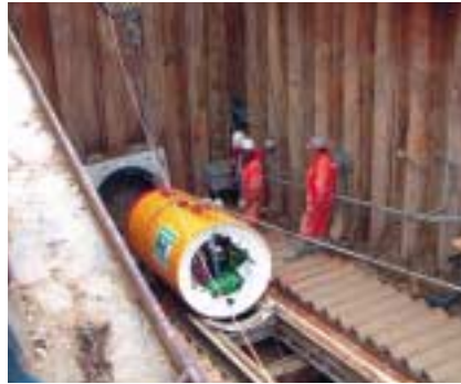
Installing the 48 in diameter casings with a microtunneller.
