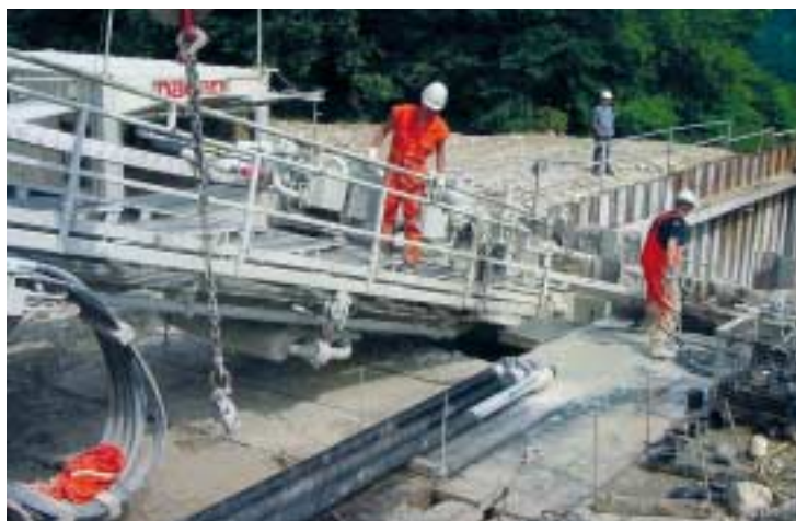
The NACAP 200 t drilling rig in operation.
