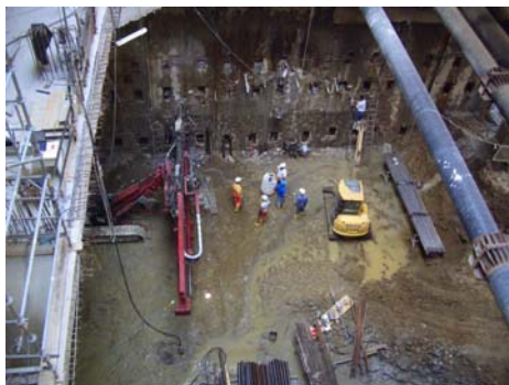
Figs 6 + 7: Drilling in progress on one of the galleries using the 10 ton EGT rig with 2m drill pipes pre-built into 9m lengths to save time in making connections to the probe.
