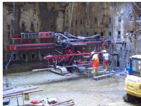
Figs 6 + 7: Drilling in progress on one of the galleries using the 10 ton EGT rig with 2m drill pipes pre-built into 9m lengths to save time in making connections to the probe.
