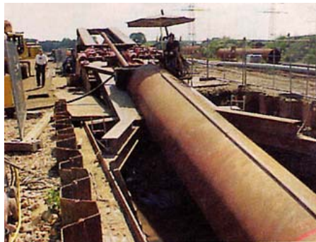
Installation of the 60-in. (1,500-mm) casing pipes
